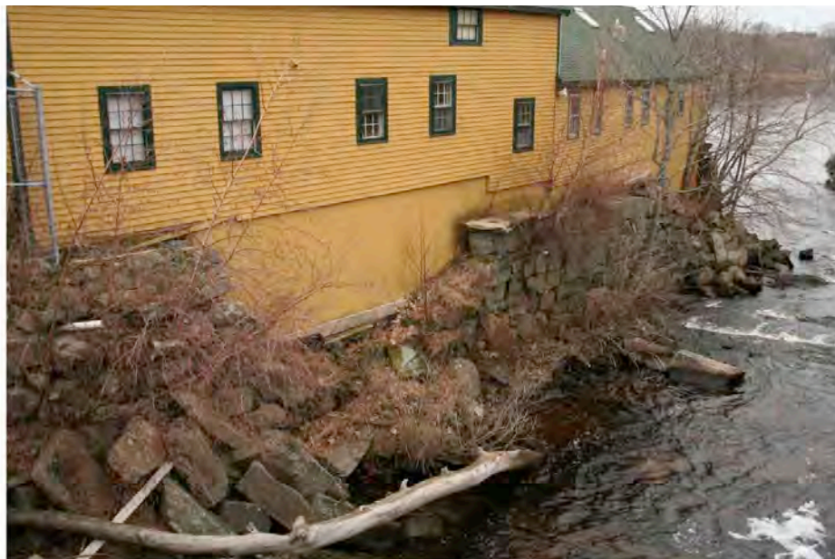
A. Downstream of dam – Left Bank of Kimball Island
