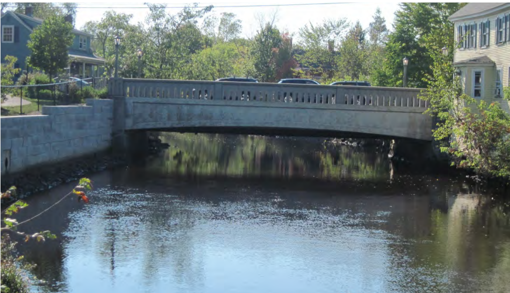
B. Looking upstream at the retaining walls at the Great Bridge.
