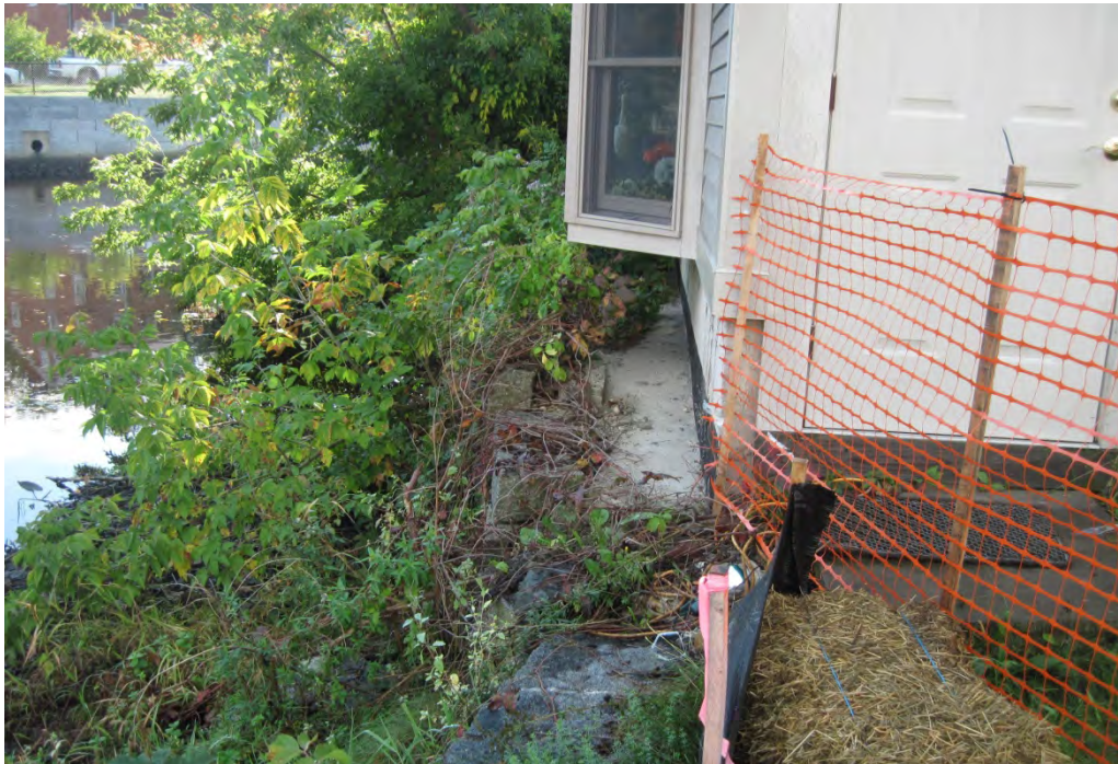
A. Concrete wall adjacent to foundation wall
