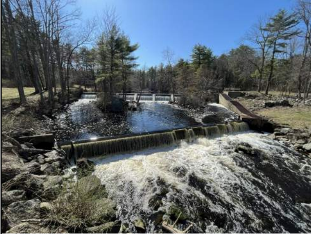
A view of Pickpocket Dam, looking upstream
