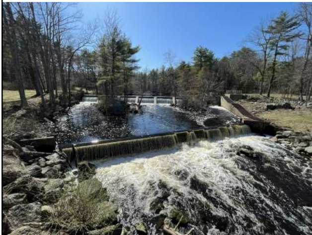
A view of Pickpocket Dam, looking upstream
