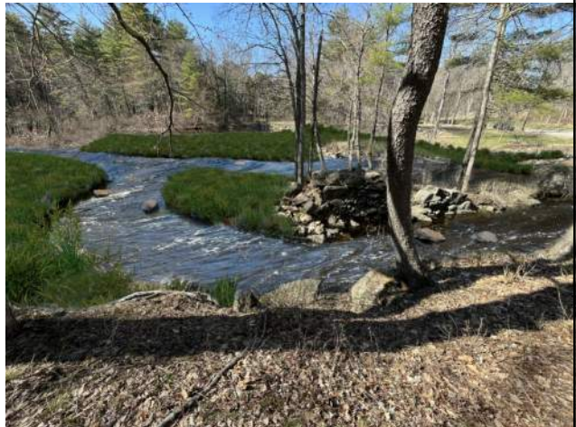
An Oblique view of Pickpocket Dam removed, looking from the right bank
