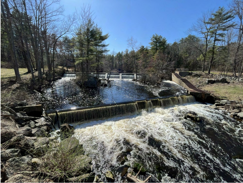
A view of Pickpocket Dam, looking upstream
