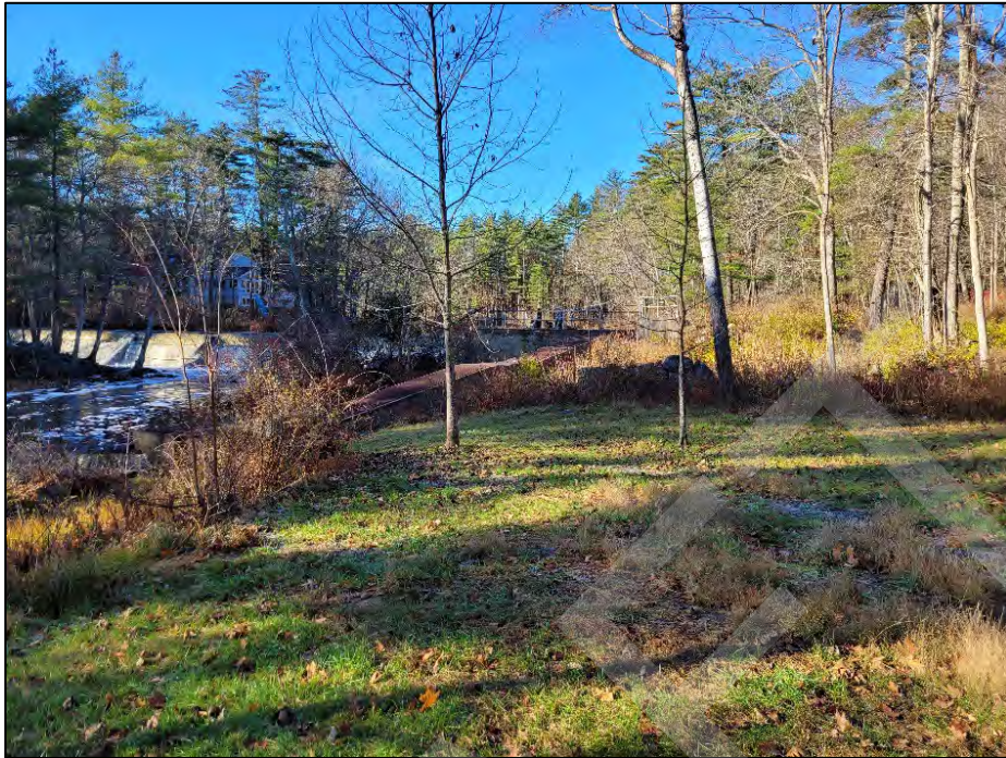
Photo No. 15.: Downstream area for the embankment left of the spillway near abandoned stone foundation.
