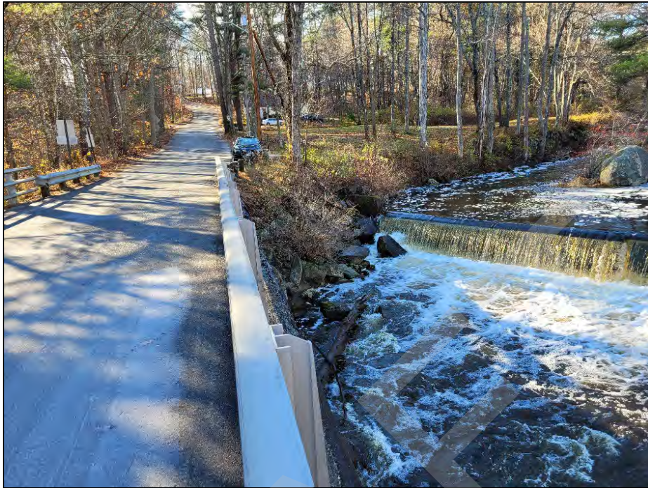
Photo No. 25.: Downstream Cross Rd. Bridge and weir just upstream of the bridge abutment.
