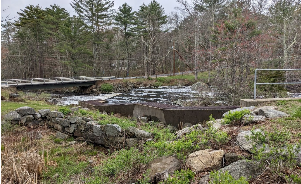
View of the Pickpocket Dam and fish ladder looking downstream from left embankment
