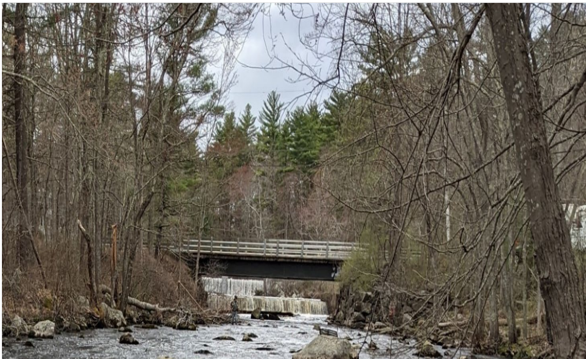
View of Pickpocket Dam looking upstream
