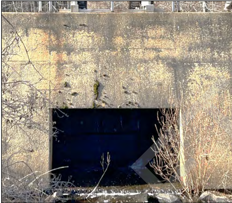
Photo No. 19.: Discharge for the low-level outlet from downstream channel. The gate is leaking from the left side of the structure.
