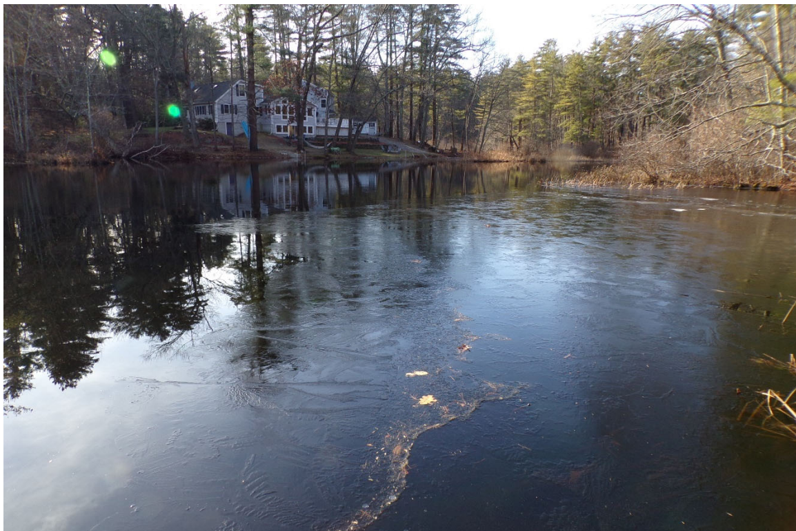
Photo 7 View west toward Exeter Reservoir impoundment above Pickpocket Dam. (Photo: VHB, December 2023.)
