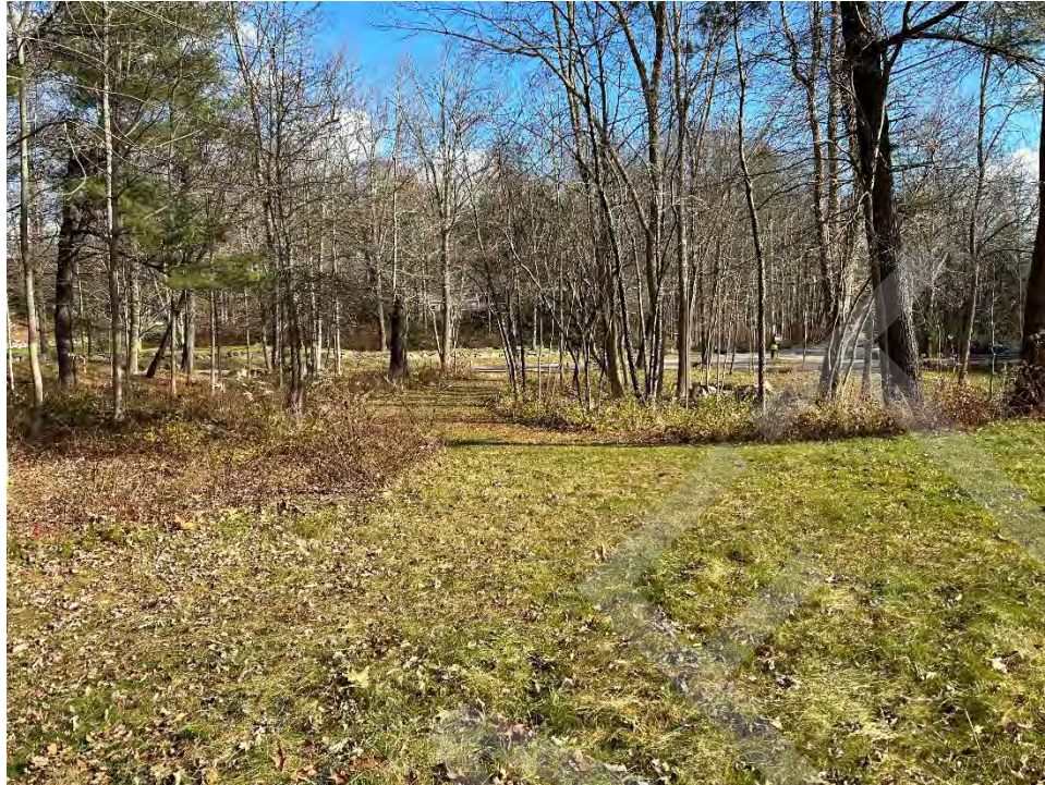
Photo No. 29.: Pathway/access point along the downstream left slope going towards Pickpocket Road near the left abutment crest.
