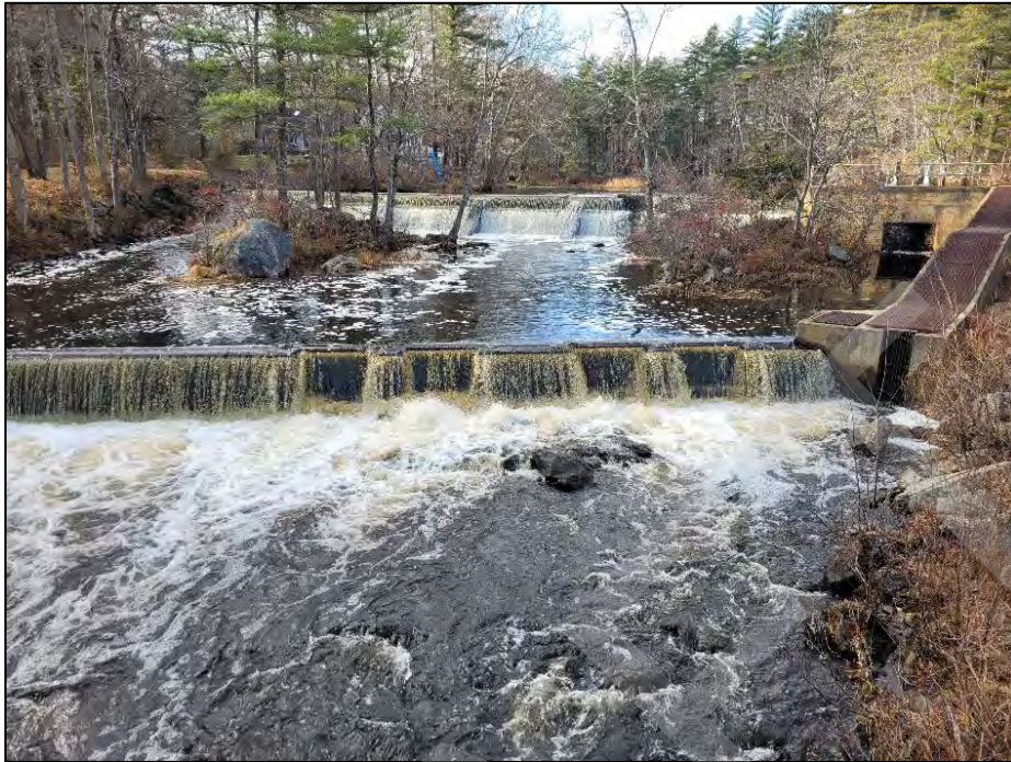
Photo No. 1.: Overview of the dam from the left bank of the downstream channel
