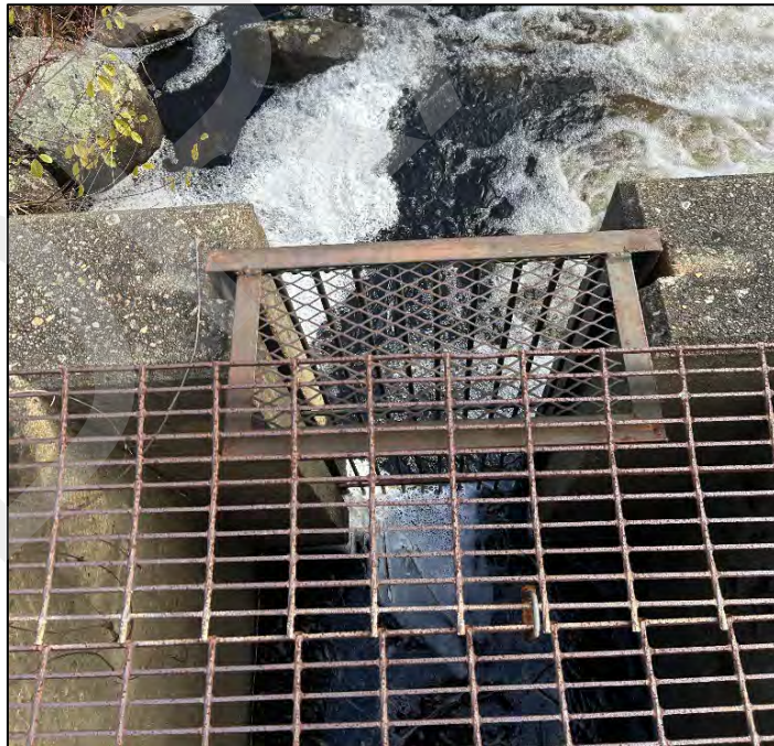
Photo No. 24.: Downstream entrance to the fish ladder.
