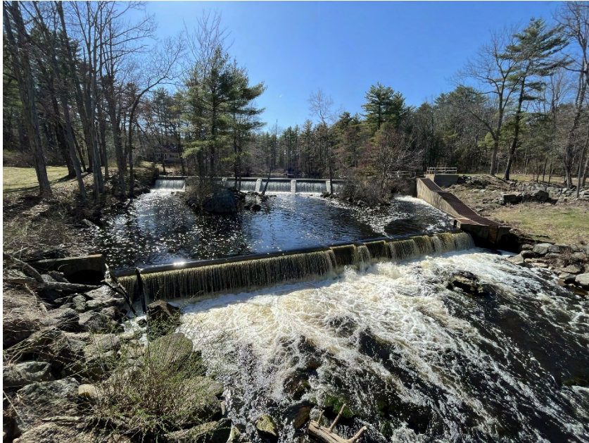
A view of Pickpocket Dam, looking upstream
