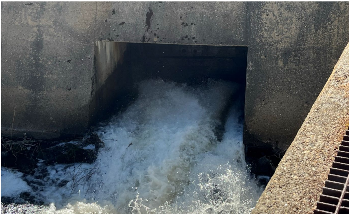
View of the low-level gate outlet of Pickpocket Dam
