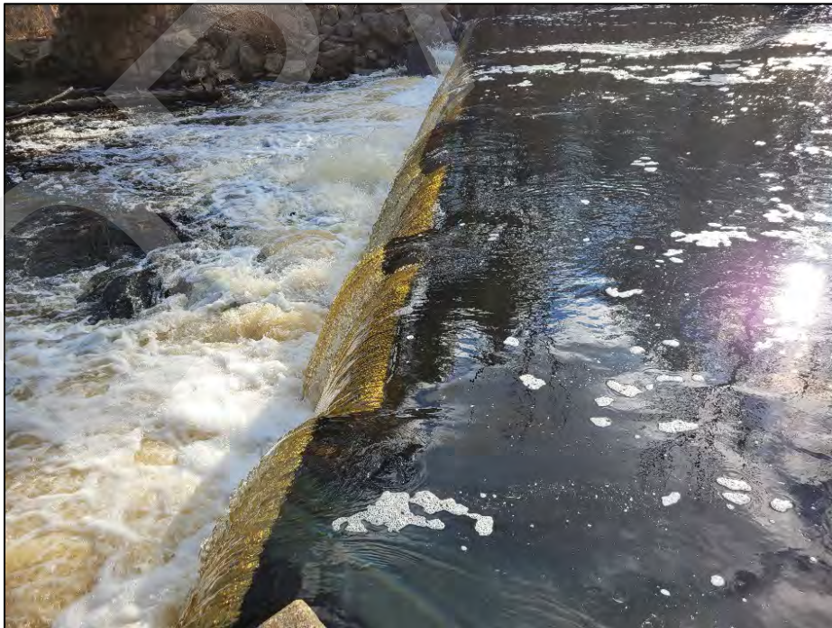
Photo No. 26.: Close up of the downstream weir crest.
