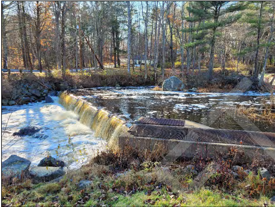
Photo No. 21.: Downstream end of fish ladder and secondary weir in the downstream channel.
