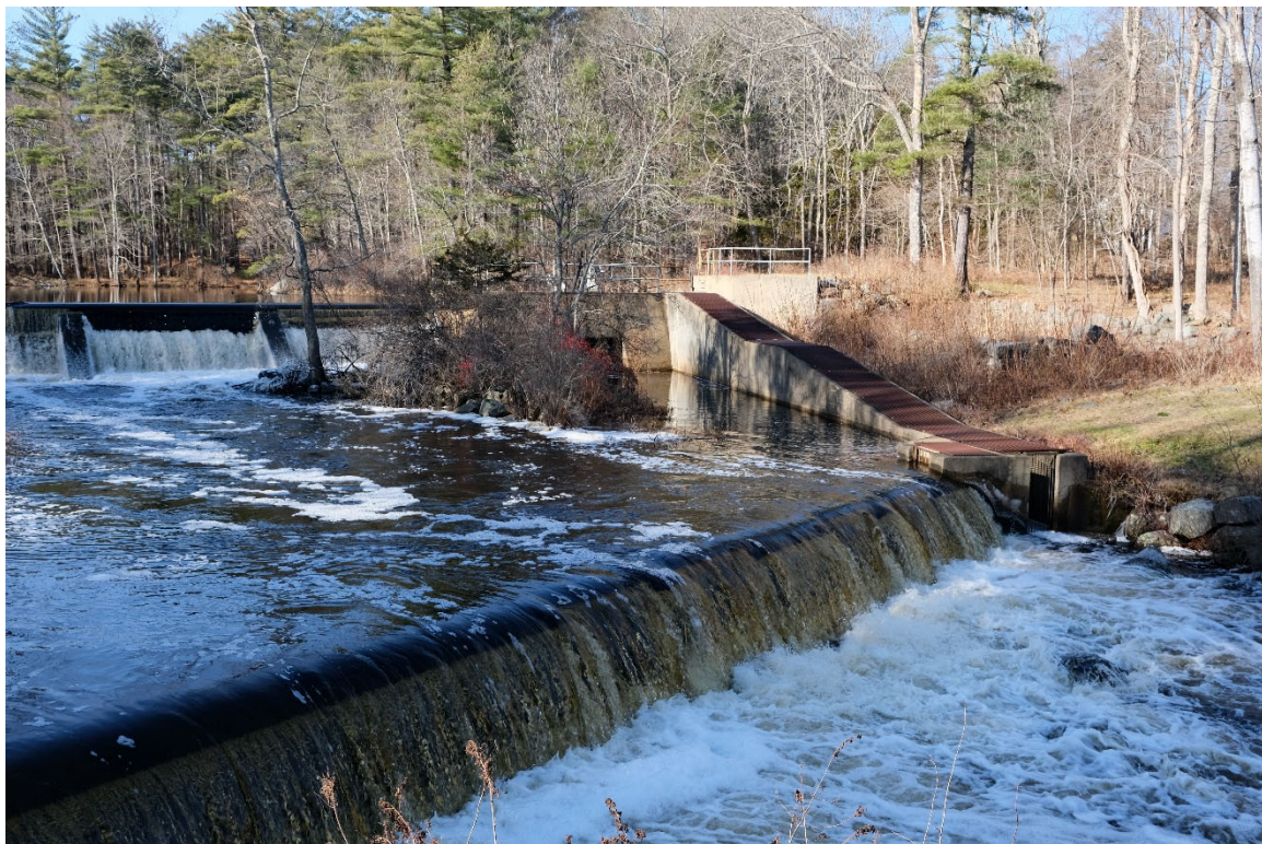
Photo 5 View northwest toward Pickpocket Dam, fish ladder, and weir. (Photo: VHB, December 2023.)
