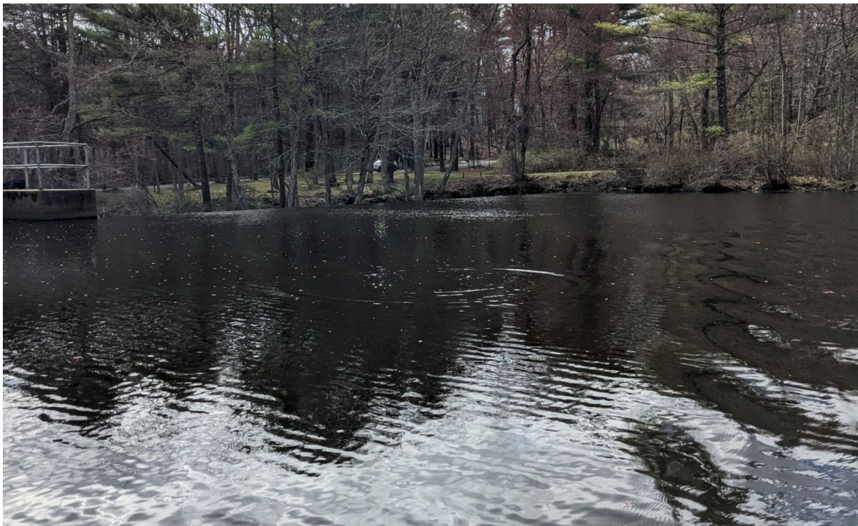
View of Pickpocket Dam looking downstream
