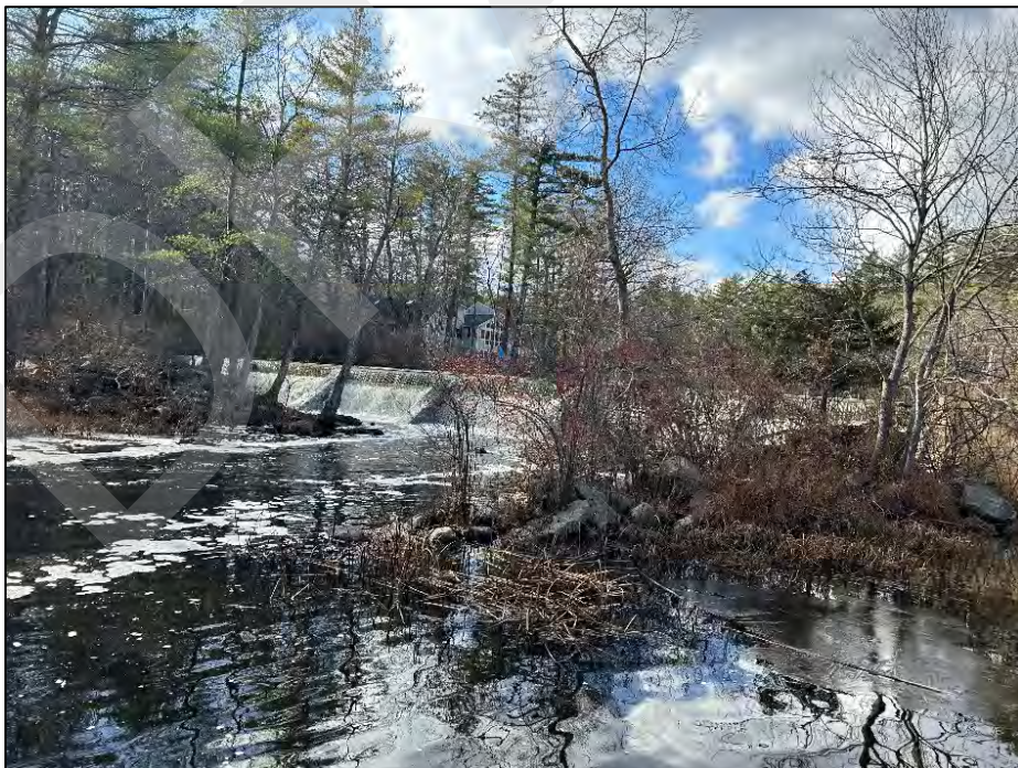
Photo No. 14.: Downstream discharge area for the low-level outlet and primary spillway from the end of the fish ladder.
