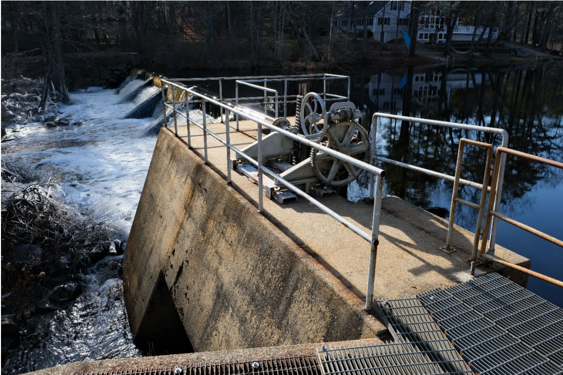
Photo 8 View south toward dam mechanicals and Pickpocket Dam. (Photo: VHB, December 2023.)
