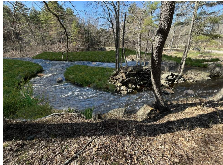
An oblique view of Pickpocket Dam removed, looking from the right bank
