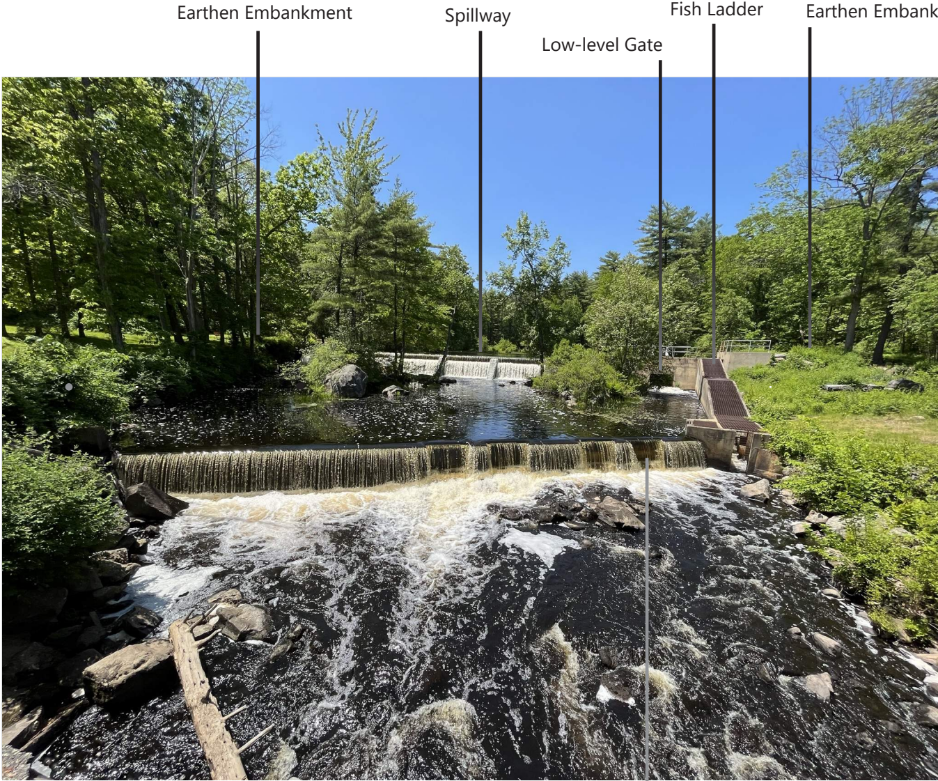
A view of the Pickpocket Dam, looking upstream from Cross Road Bridge
