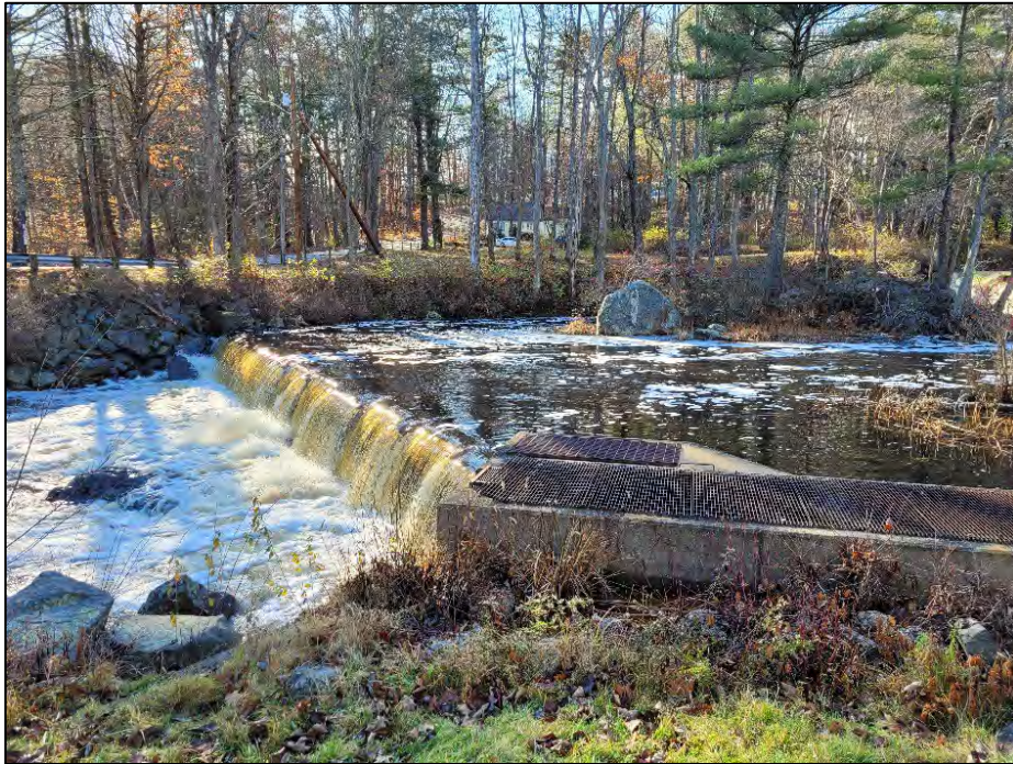
Photo No. 21.: Downstream end of fish ladder and secondary weir in the downstream channel.
