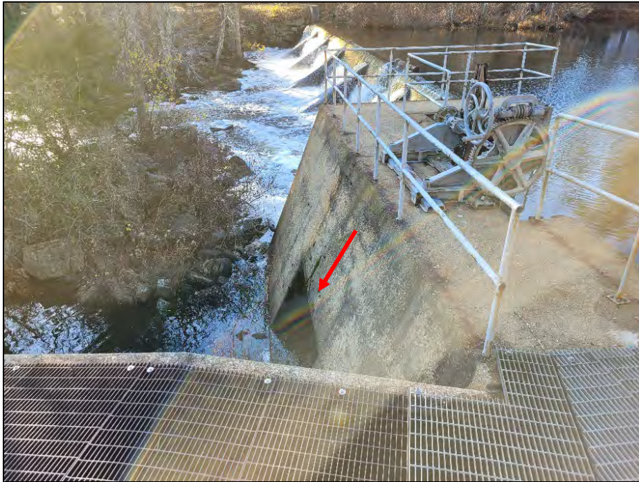
Photo No. 7.: Overview of the downstream side of the low-level outlet discharge (arrow) and the spillway.
