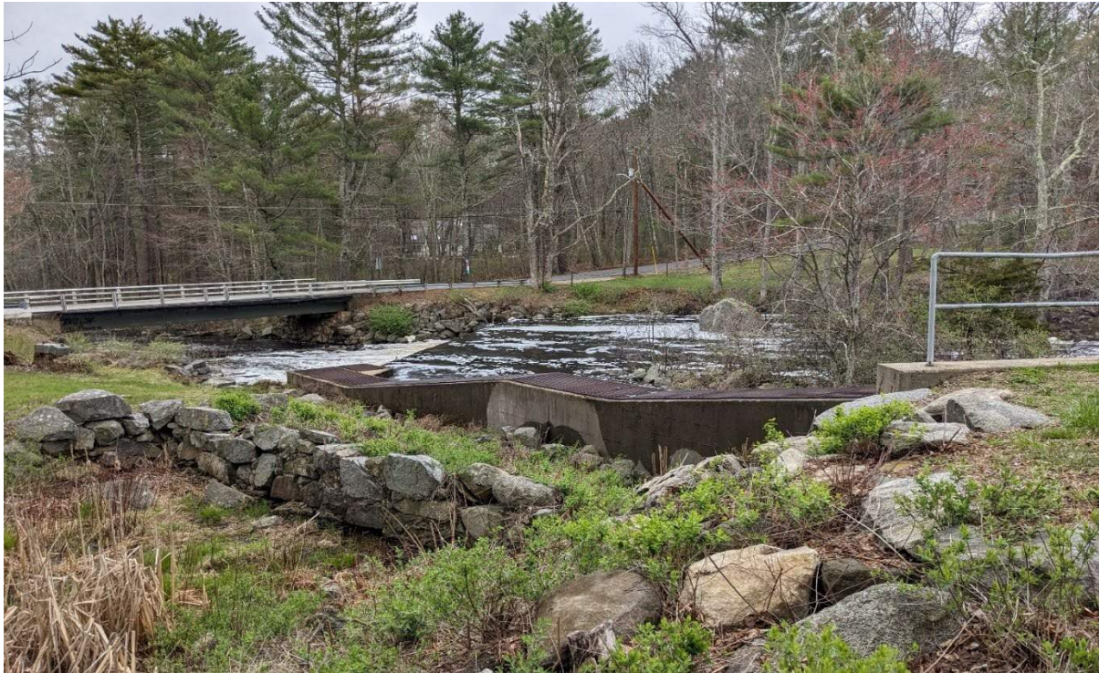
View of the Pickpocket Dam and fish ladder looking downstream from left embankment
