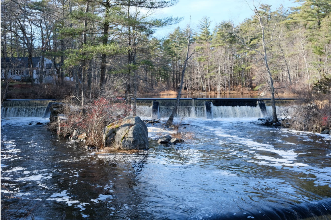
Photo 4 View west toward Pickpocket Dam. (Photo: VHB, December 2023.)
