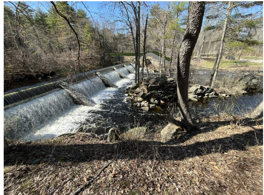
An oblique view of Pickpocket Dam primary spillway with Alternative 1, looking from the right bank
