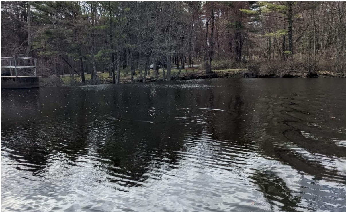
View of Pickpocket Dam looking downstream
