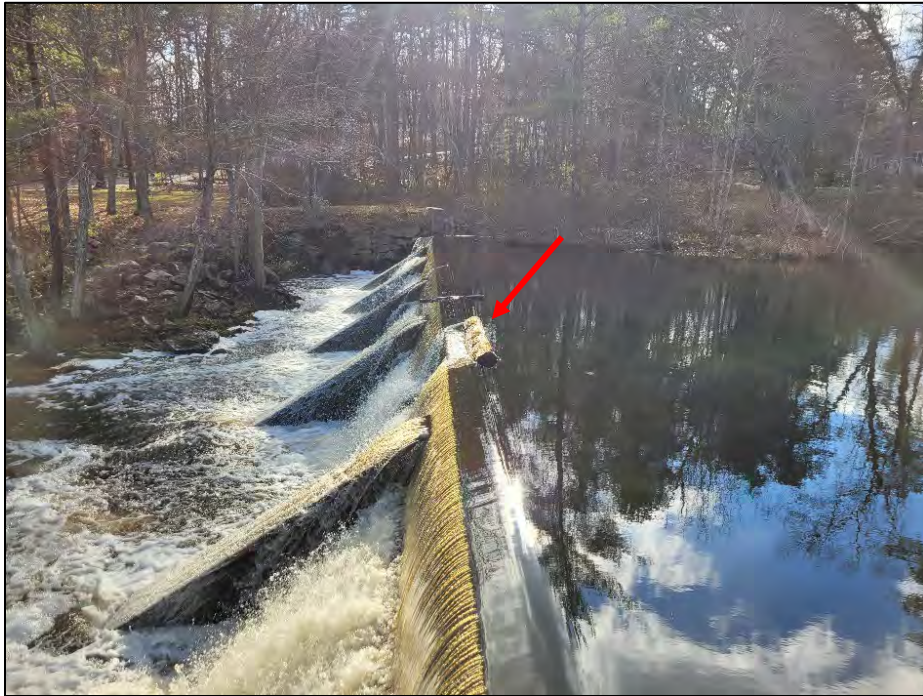
Photo No. 3.: View of the primary spillway crest. Note the timber log debris (arrow) on the crest.
