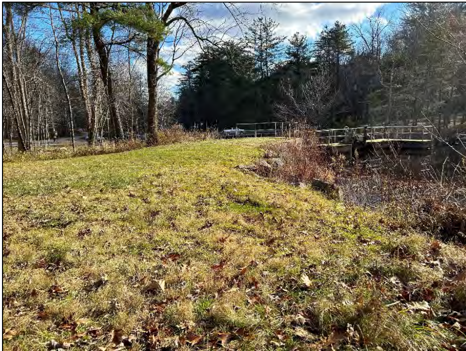
Photo No. 4.: View of the embankment left of the spillway.
