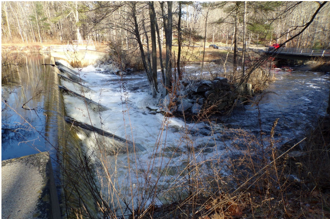
Photo 3 View north-northeast toward Pickpocket Dam. (Photo: VHB, December 2023.)
