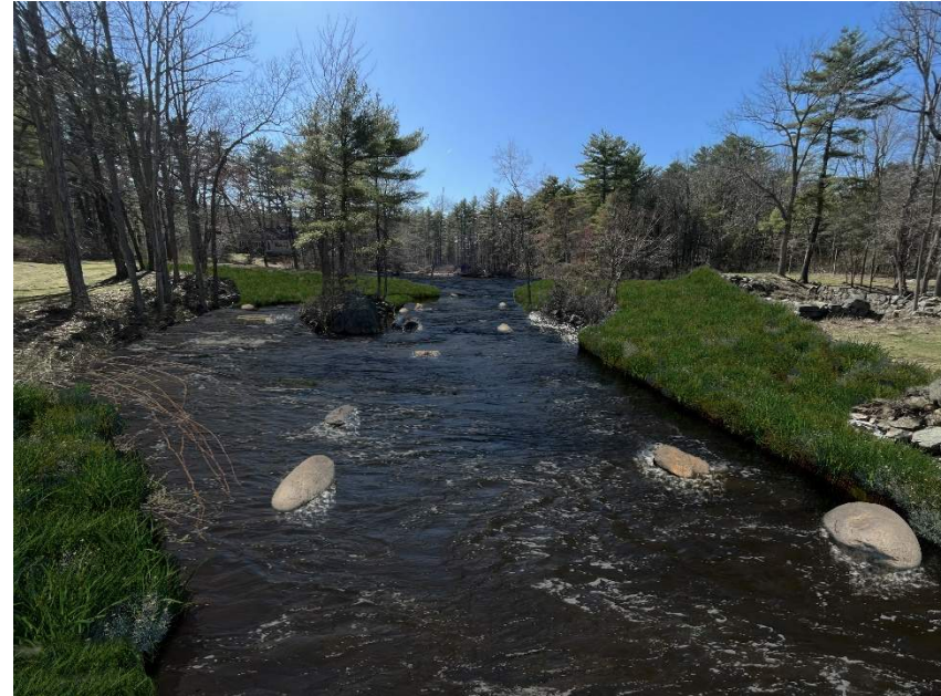
A view of Pickpocket Dam removed, looking upstream
