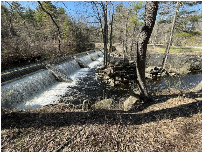
An oblique view of Pickpocket Dam primary spillway, looking from the right bank
