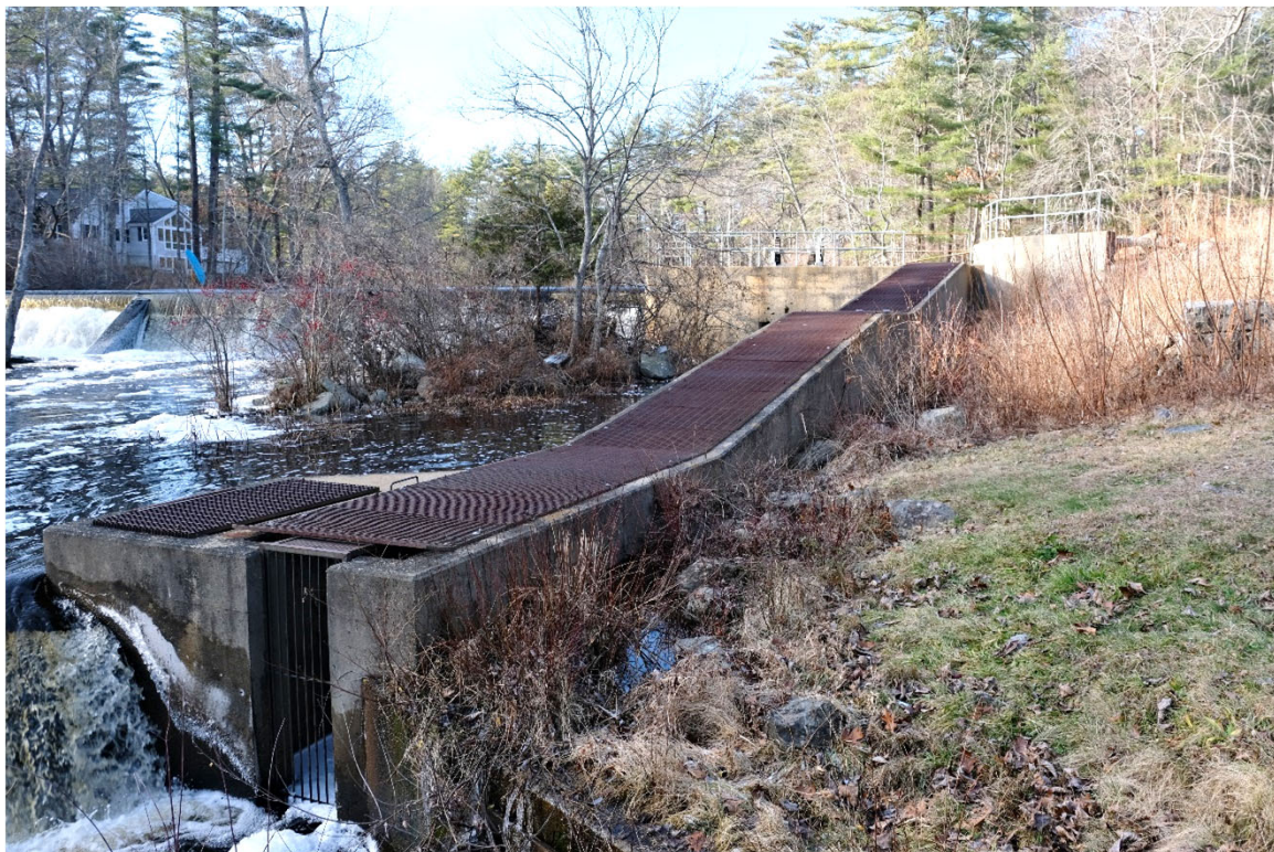
Photo 9 View west-southwest toward fish ladder. (Photo: VHB, December 2023.)
