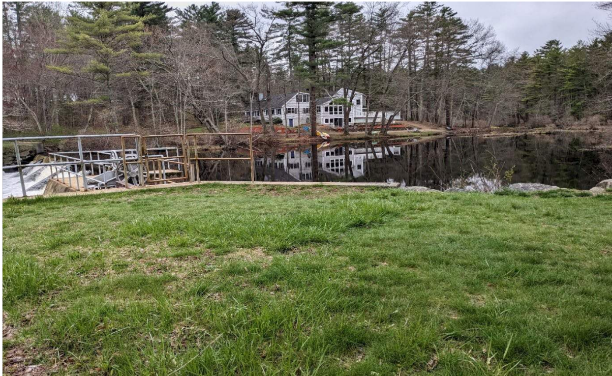
View of Pickpocket Dam looking upstream at the impoundment
