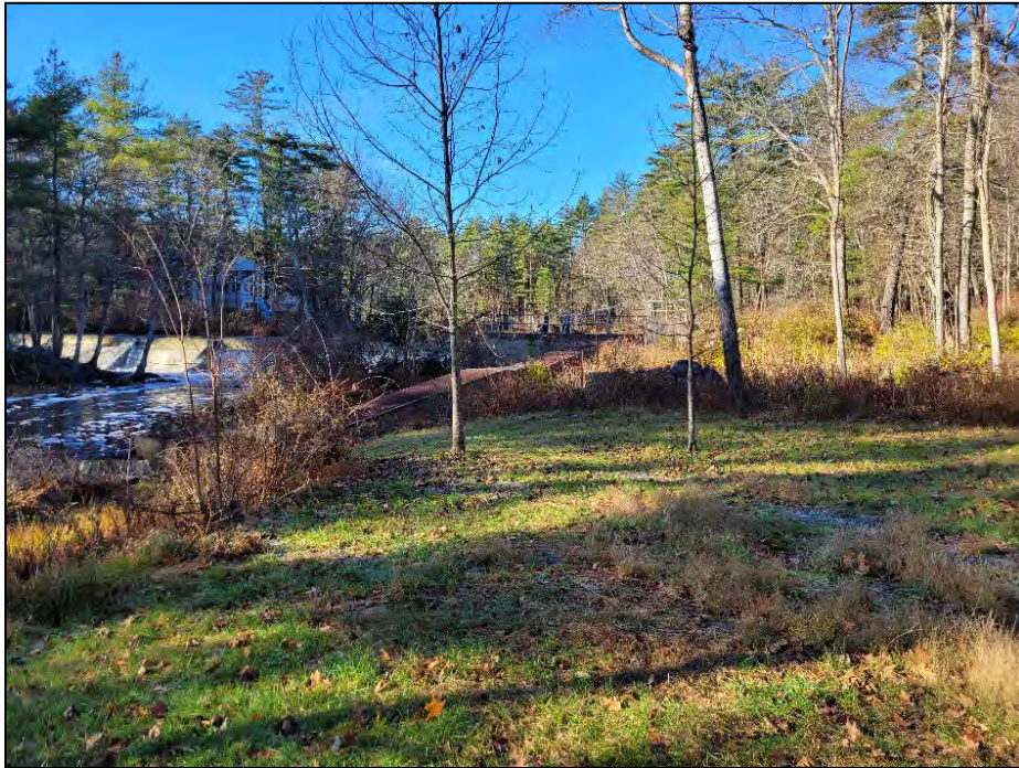
Photo No. 15.: Downstream area for the embankment left of the spillway near abandoned stone foundation.
