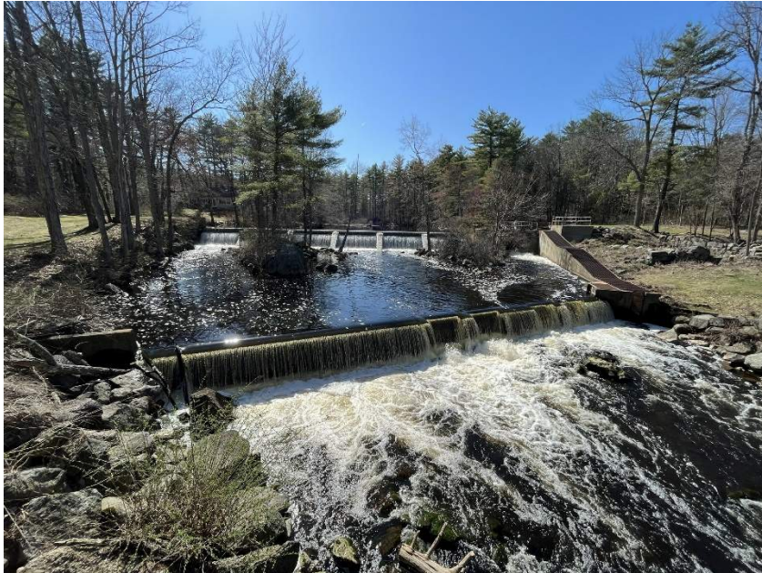
A view of Pickpocket Dam, looking upstream
