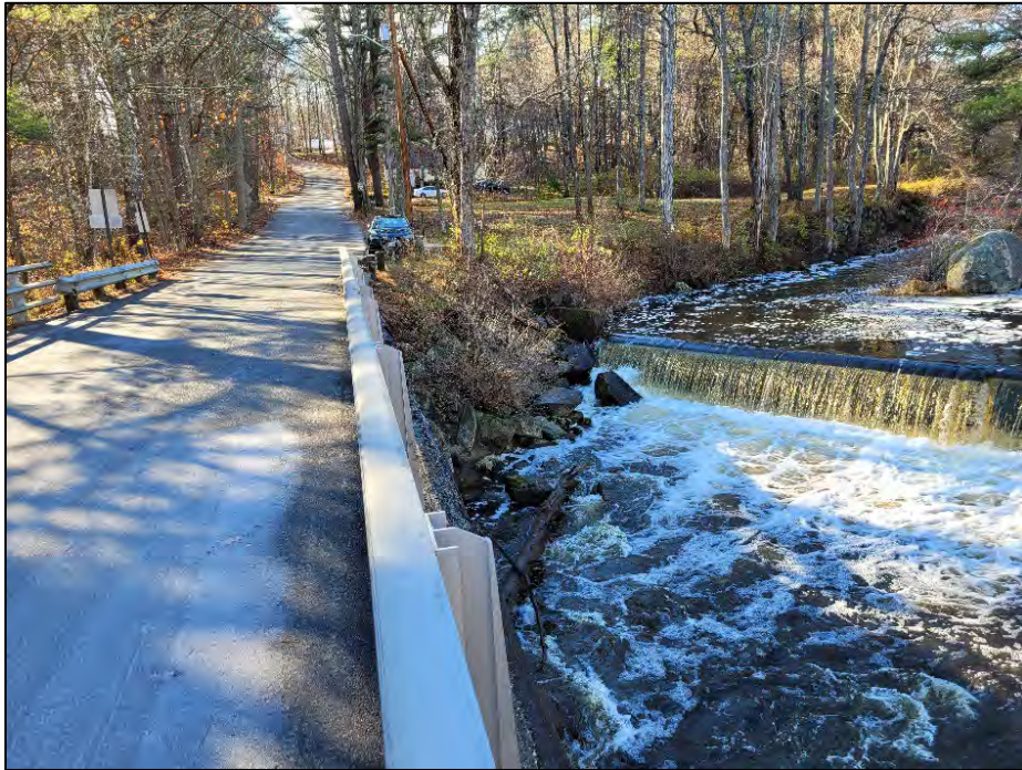
Photo No. 25.: Downstream Cross Rd. Bridge and weir just upstream of the bridge abutment.
