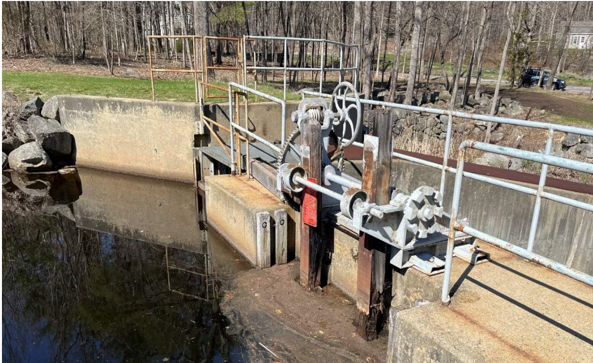
View of the low-level gate entrance of Pickpocket Dam
