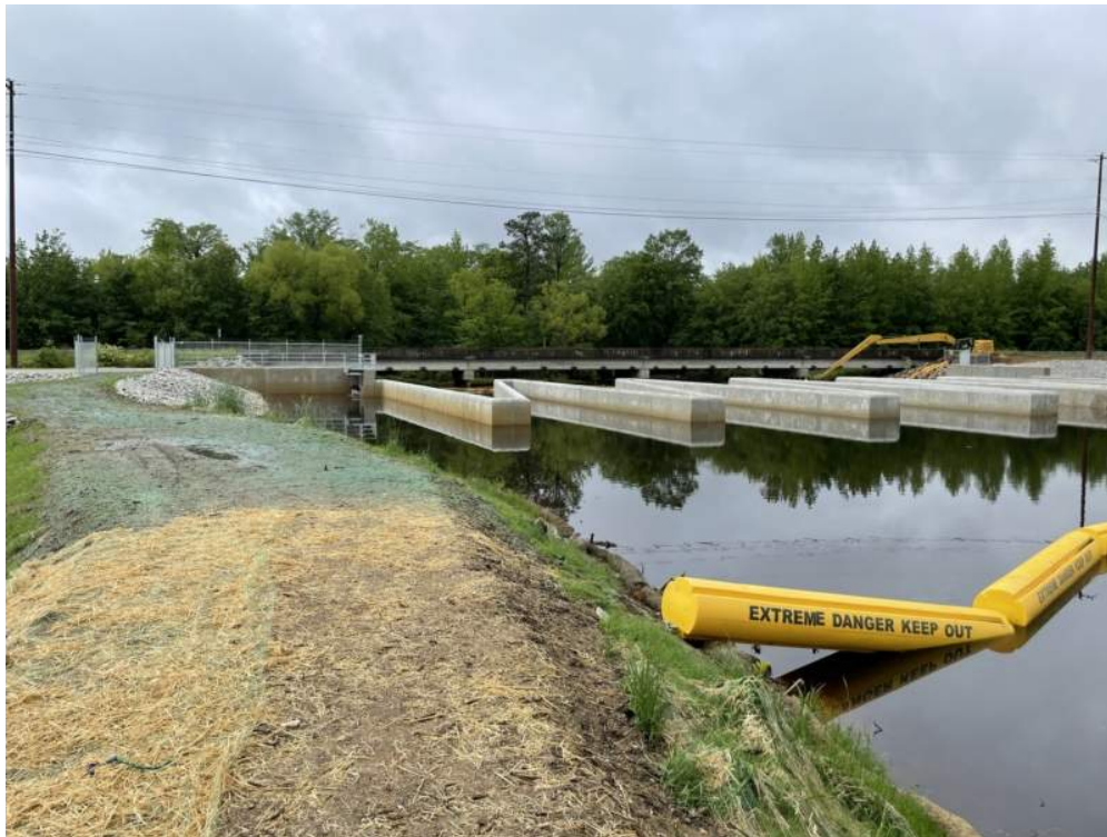
Figure 2.3-2: Example Picture of Labyrinth Spillway
