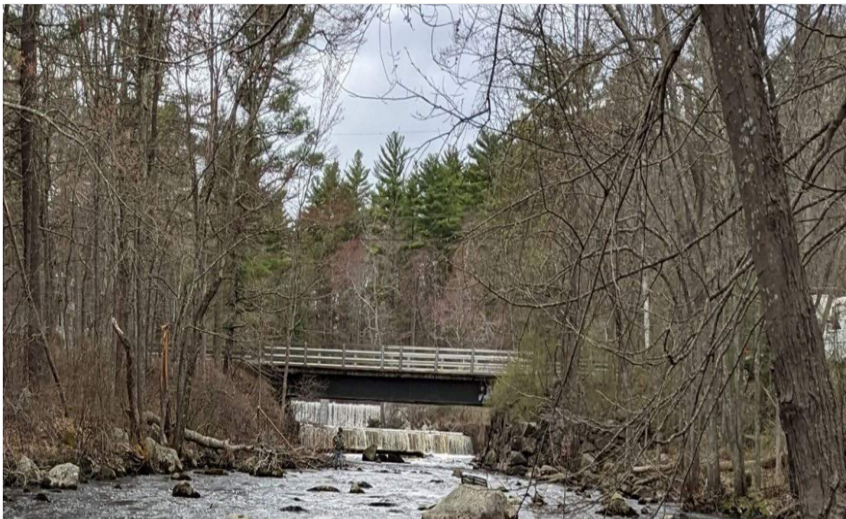
View of Pickpocket Dam looking upstream
