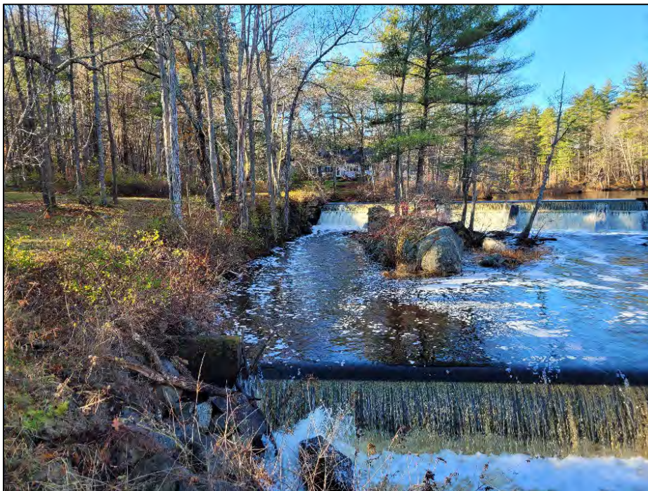
Photo No. 6.: Right side of the downstream channel wall and embankment right of the spillway from downstream bridge. Note the vegetated island within the downstream channel.
