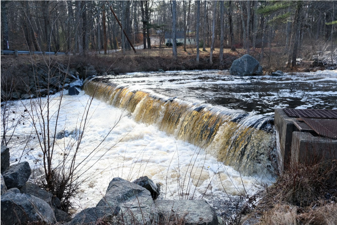
Photo 10 View south toward weir and base of fish ladder. (Photo: VHB, December 2023.)
