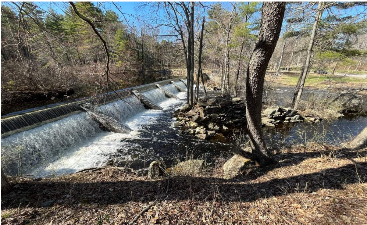
Side view of Pickpocket Dam and spillway looking north, from right bank
