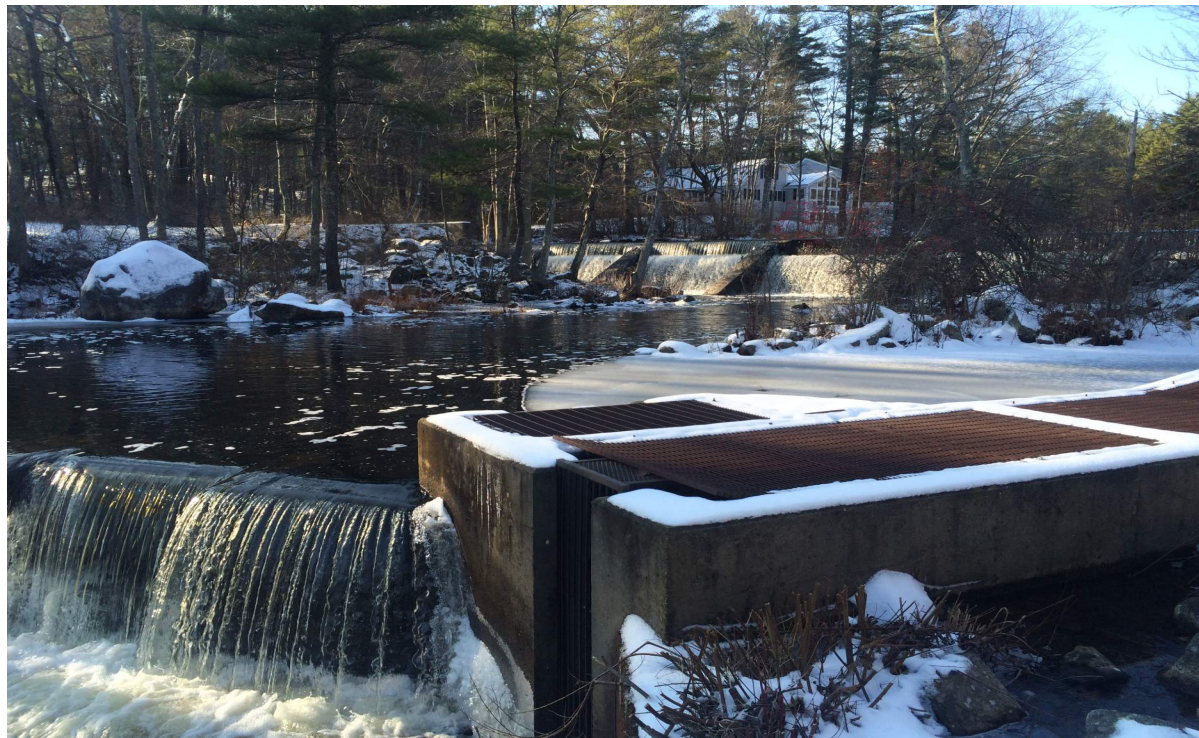
View of the fish ladder downstream of Pickpocket Dam at training weir.
