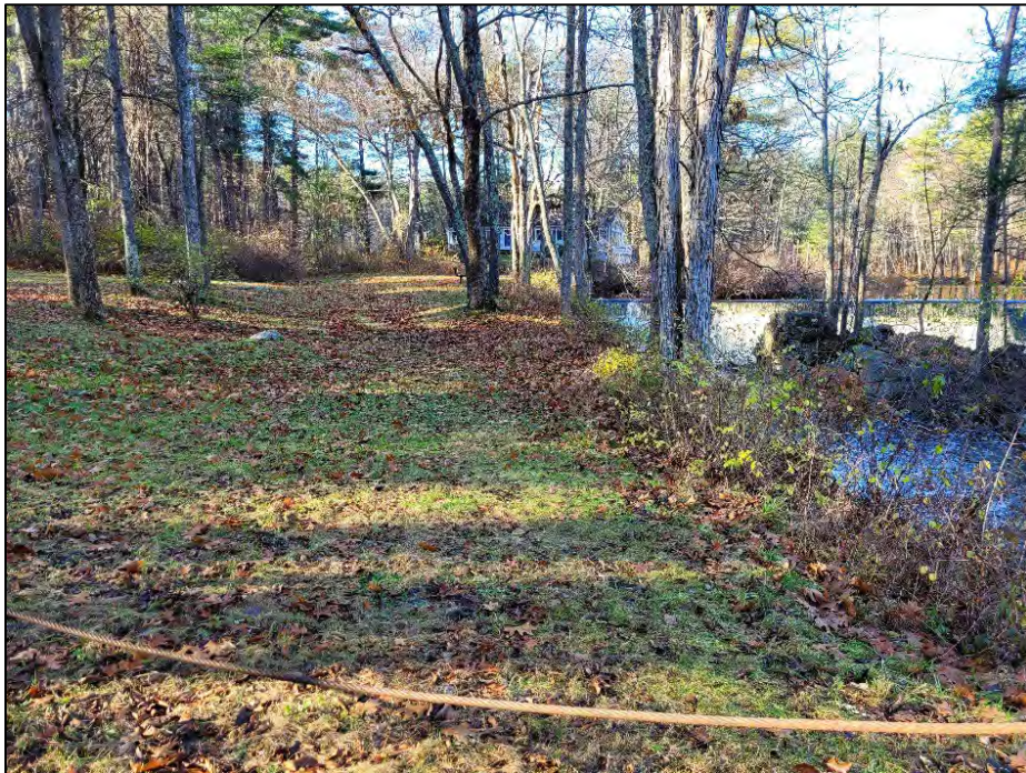
Photo No. 8.: Right abutment from the downstream access road looking upstream.
