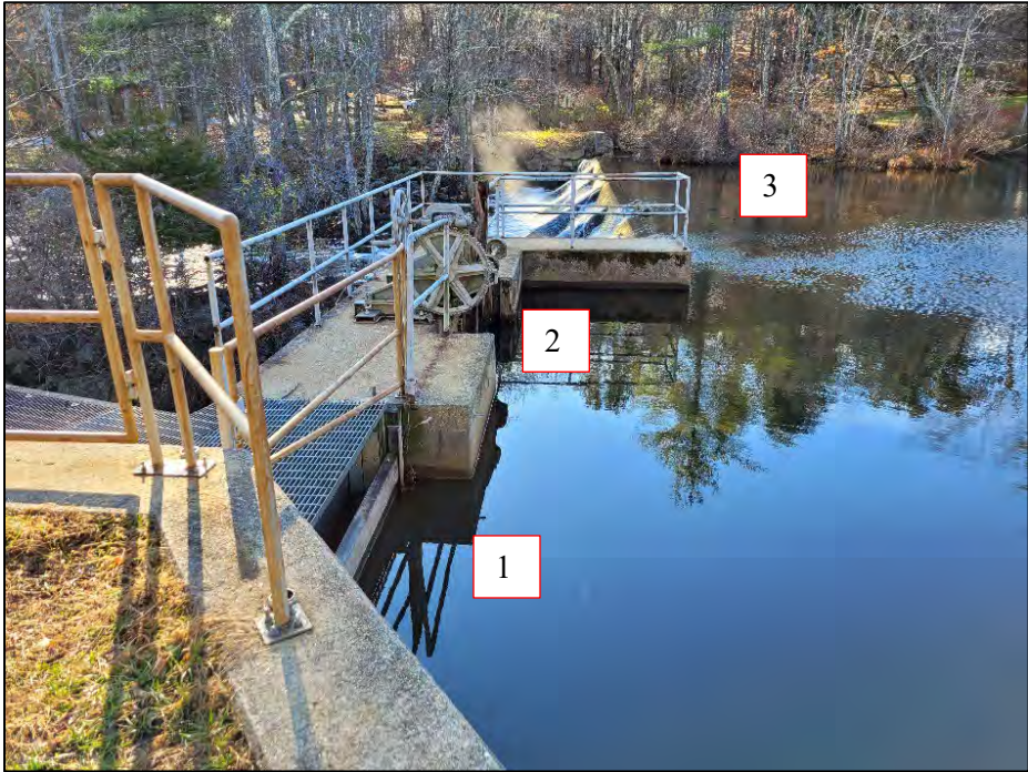
Photo No. 2.: Overview of the fishway entrance (1), low-level outlet entrance (2), and primary spillway (3) from the left training wall.
