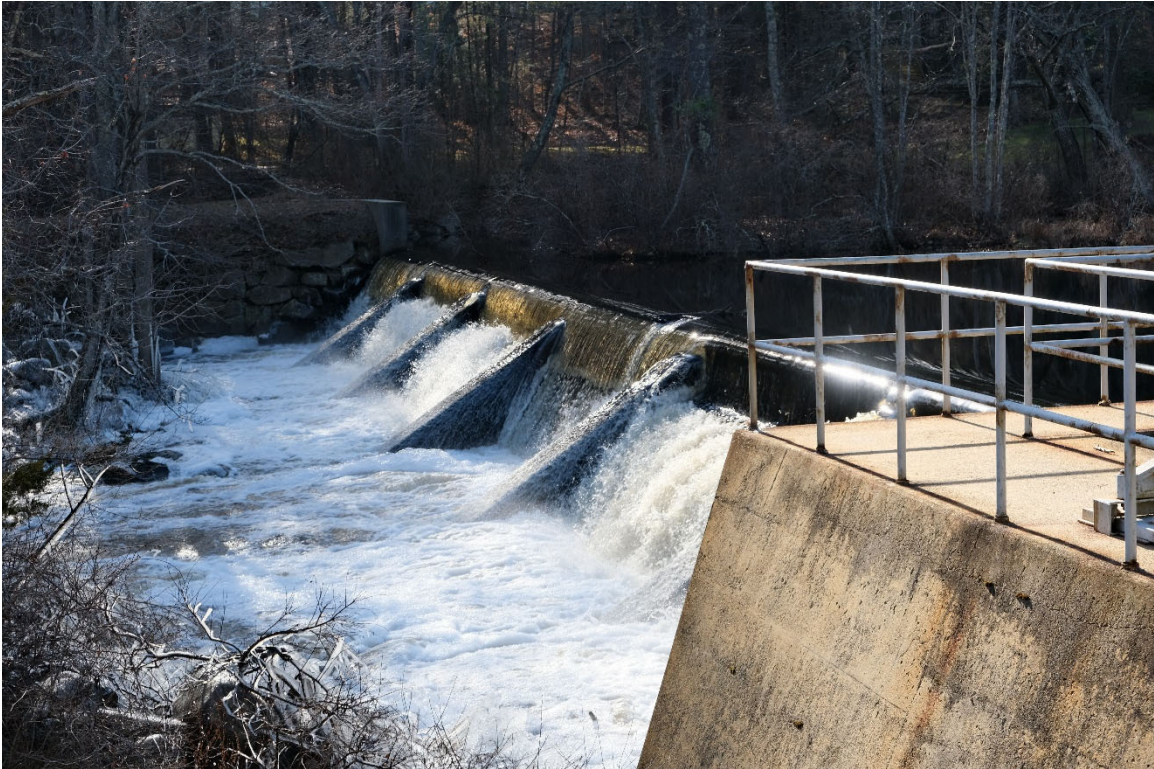
Photo 6 View south-southwest toward Pickpocket Dam. (Photo: VHB, December 2023.)
