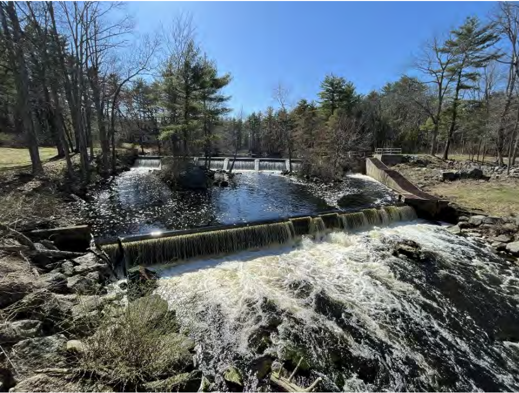
A view of Pickpocket Dam, looking upstream
