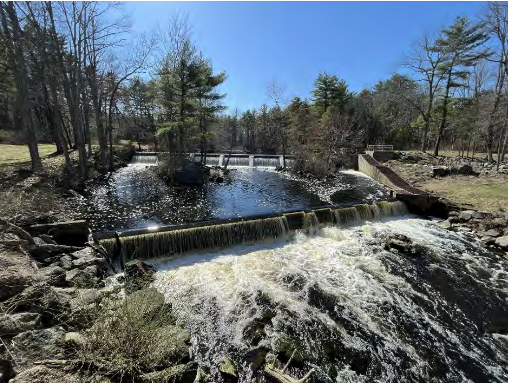
A view of Pickpocket Dam, looking upstream
