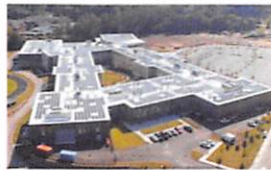
City of Dover Dover High School, Indoor Pool, CMNH 1 MW (2018-9)
