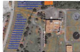
City of Concord Solar Thermal + Waste Water Treatment Plant 720 kW (2015, 2020)
