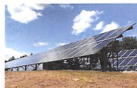
City of Lebanon Wastewater Treatment Facility + 6 Rooftops 836 kW (2019)
