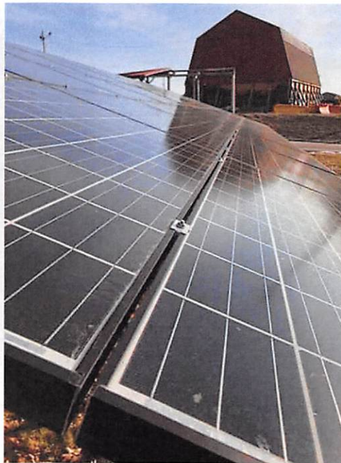
5.0 Modules and Racking - General photos
