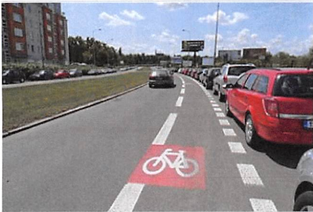
Počernická street in Prague used to be four lanes wide. In 2010s, it got two parking lanes and bicycle lanes on each side of the road
