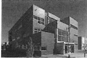
Manchester Municipal Complex Manchester, NH 2012 - New, 143,000 SF, $38.0M Police HQ, DPW Administration Building and Fleet Maintenance Building 2013 Honor Award (New Hampshire AIA) (left, above and right)
