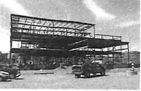
Beverly Police Station Beverly, MA Under Construction - New, 32,600 SF, $23.0M
