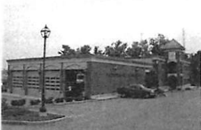
Shrewsbury Fire Headquarters Shrewsbury, MA 2007 - New, 16,000 SF, $4.6M
