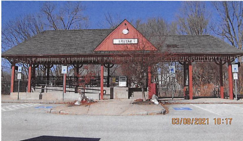
Front of Platform—looking north
