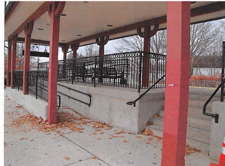
Access to high platform
