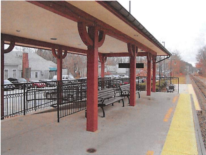
High platform trackside looking west
