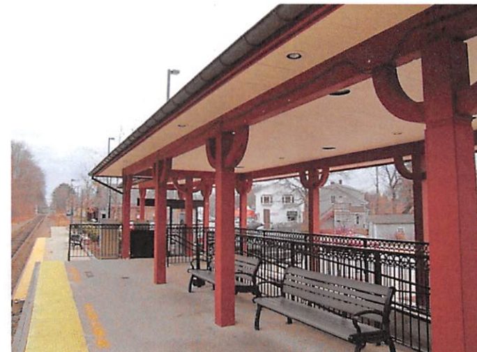
High platform trackside looking East
