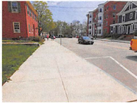
Improved sidewalks along Front Street
