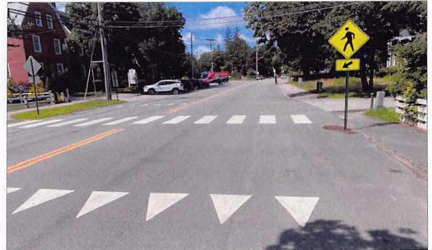
High visibility crosswalk markings installed on Front Street in 2023
