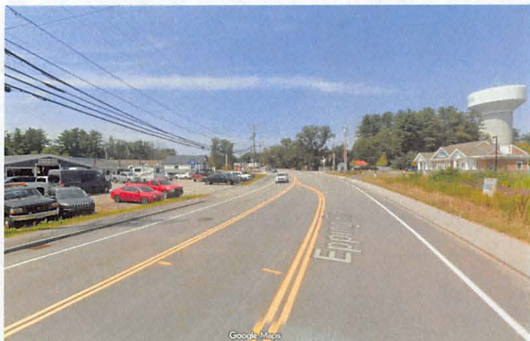
Epping Road Existing Conditions
