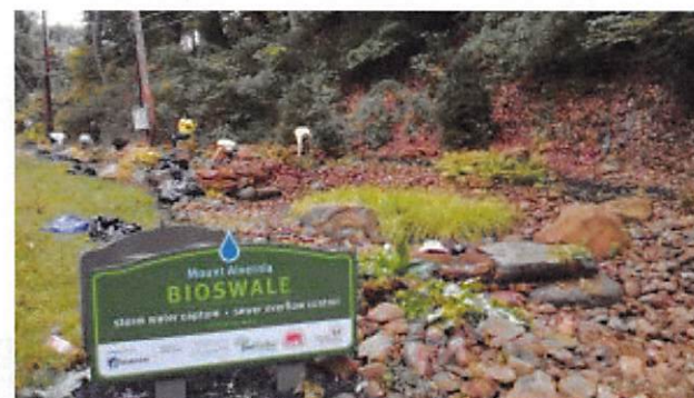
Bioswale to reduce the negative impacts of stormwater ( https://pittsburghgreenstory.com/zaheen-hussain/ )
