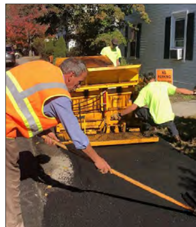
Highway Team members Perkins, Batchelder & McCallum use the sidewalk paver on Elm Street.
