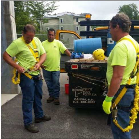
Safety First! Water/Sewer team members Dalton and Bugbee don climbing harnesses with oversight from Foreman Souza before ascending Epping Road Tank.
