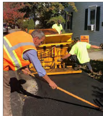
Highway Team members Perkins, Batchelder & McCallum use the sidewalk paver on Elm Street.
