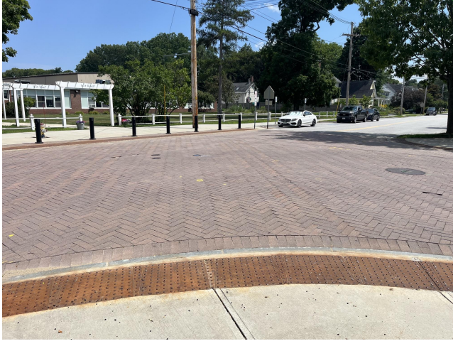
Raised intersection at train station parking area
