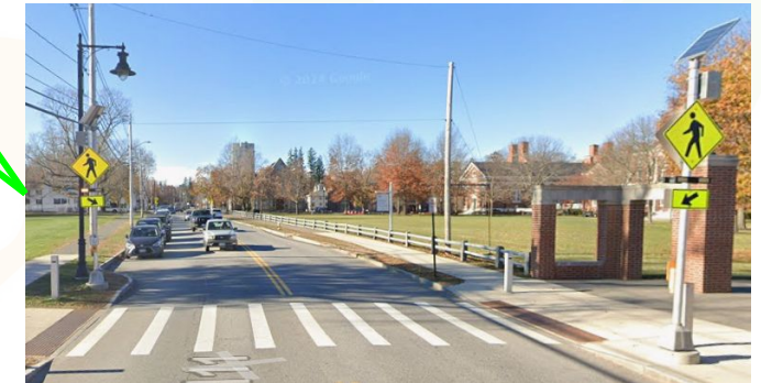
Flashing beacons (RRFB) at mid-block crossings
