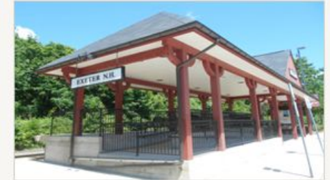
Mini-high platform — the upgrade starting point
