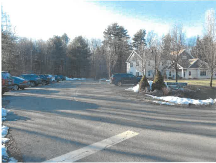
Subject Property – Paved Drive & Office Building Looking West from White Oak Drive - (2/24)
