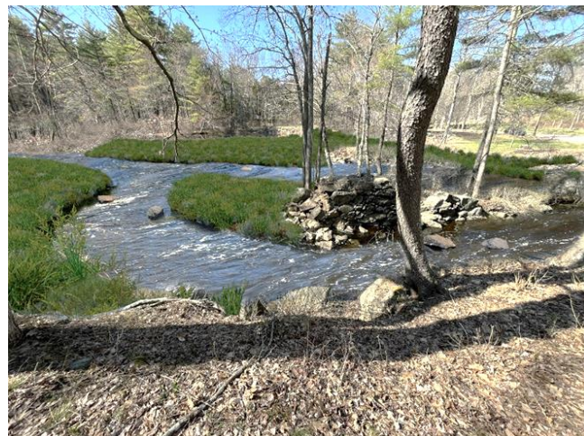
An oblique view of Pickpocket Dam removed (Alternative 4), looking from the right bank.
